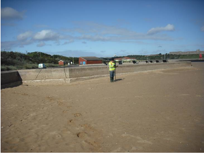
Plate 1 – Survey photograph 1bSS4_20110916_N4.JPG
