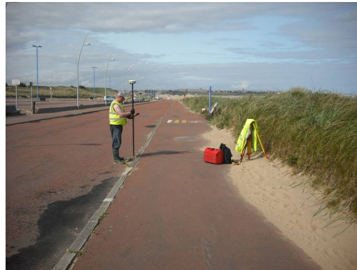
Plate 5 – Survey photograph 1bSS9_20110916_N1.JPG
